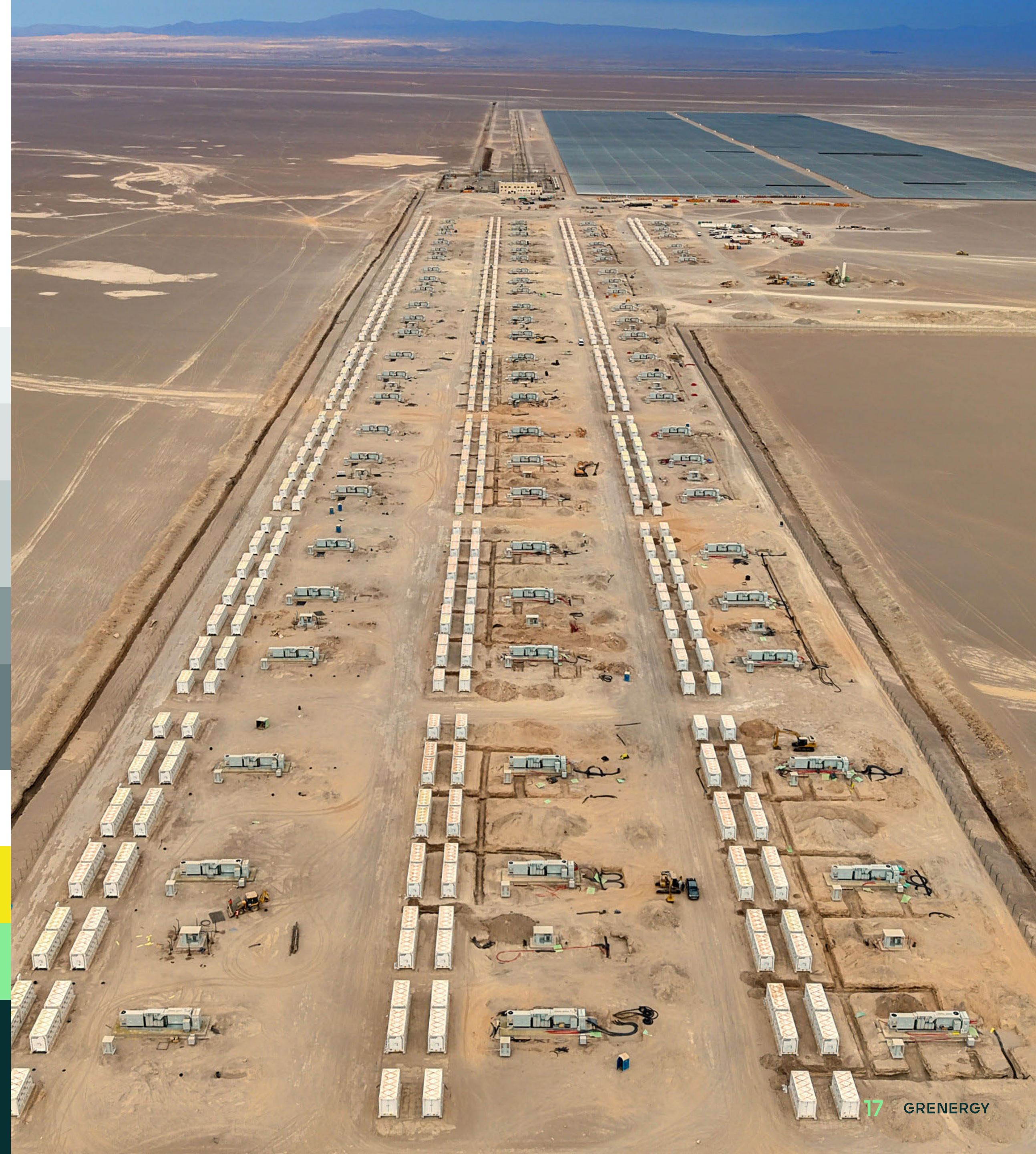
Elena project under construction phase
