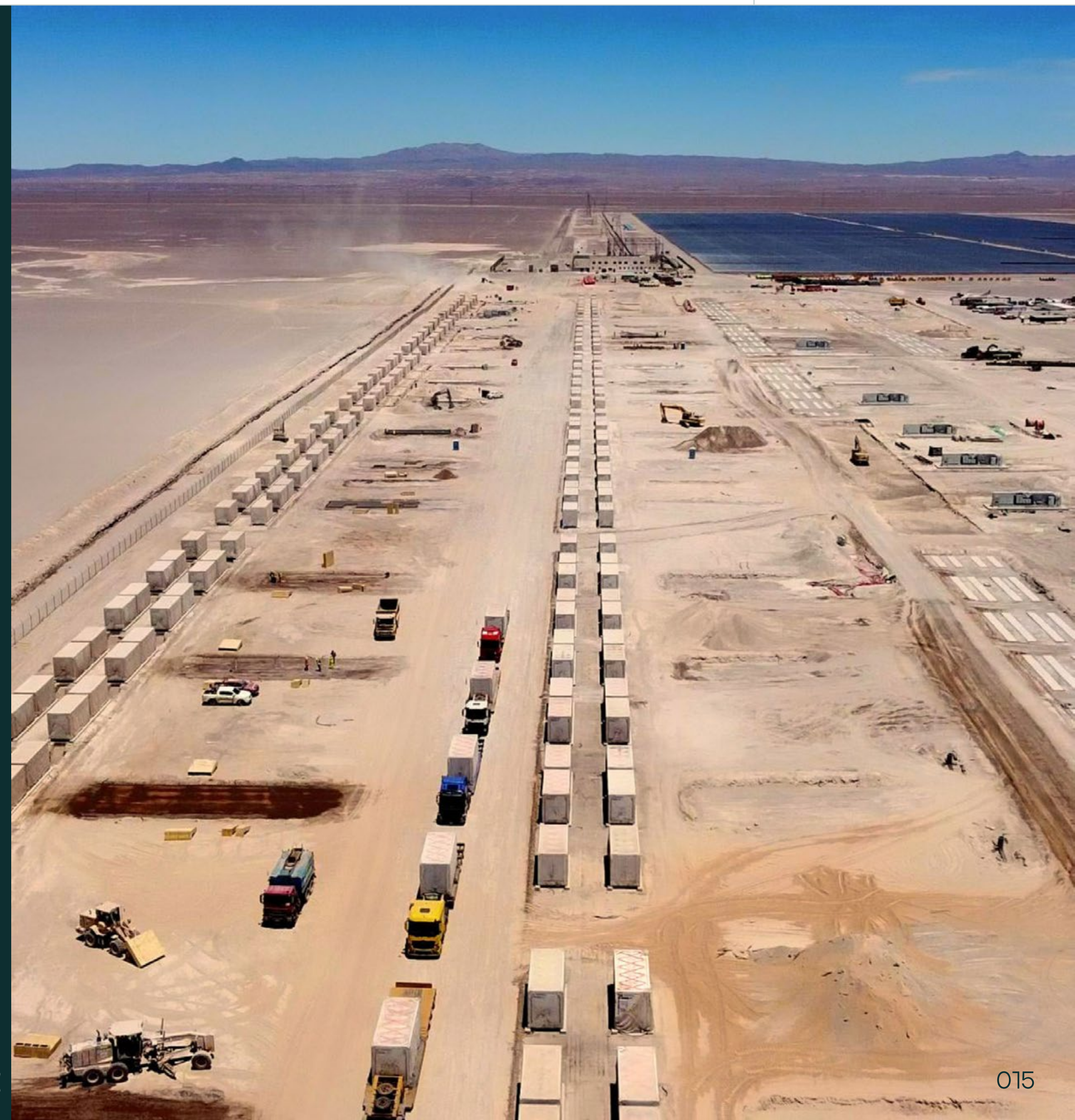
Elena 446 MW + 3.5 GWh hybrid plant, Chile
