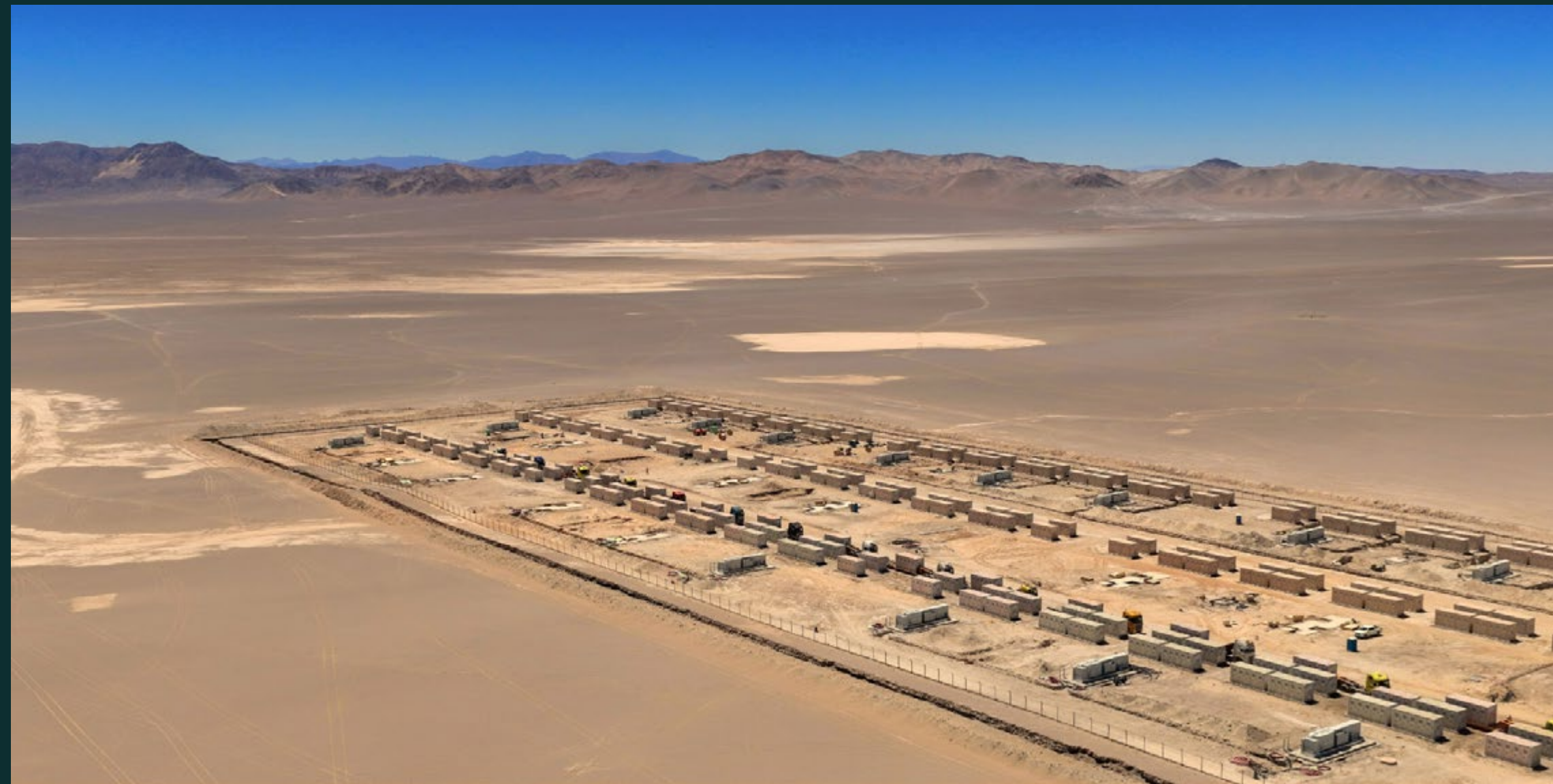
Elena 446 MW + 3.5 GWh hybrid plant, Chile
