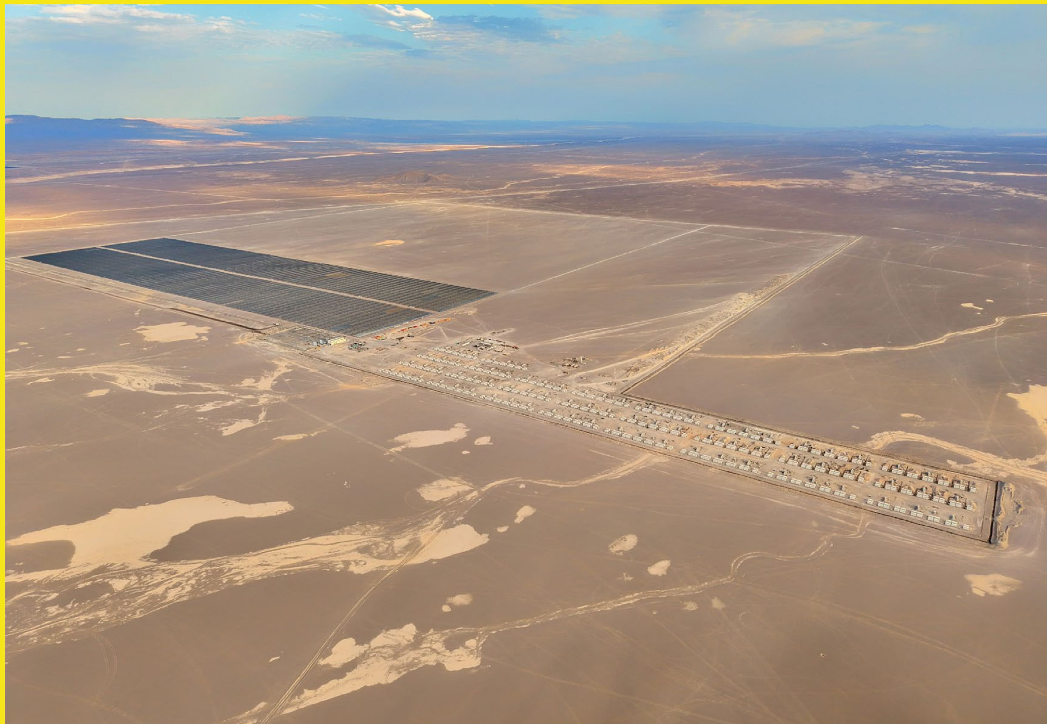
Elena 446 MW + 3.5 GWh hybrid plant, Chile
