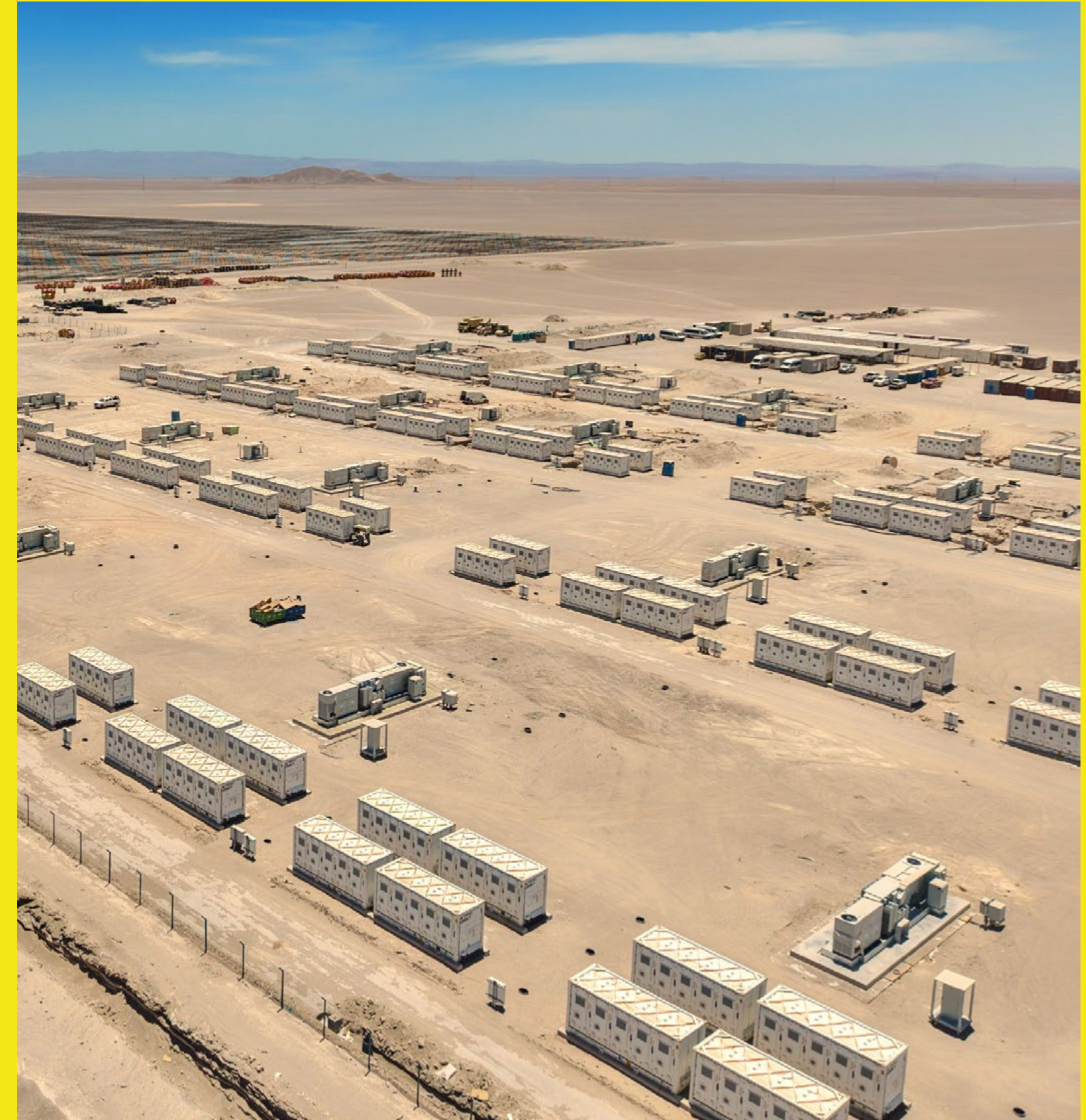
Elena 446 MW + 3.5 GWh hybrid plant, Chile
