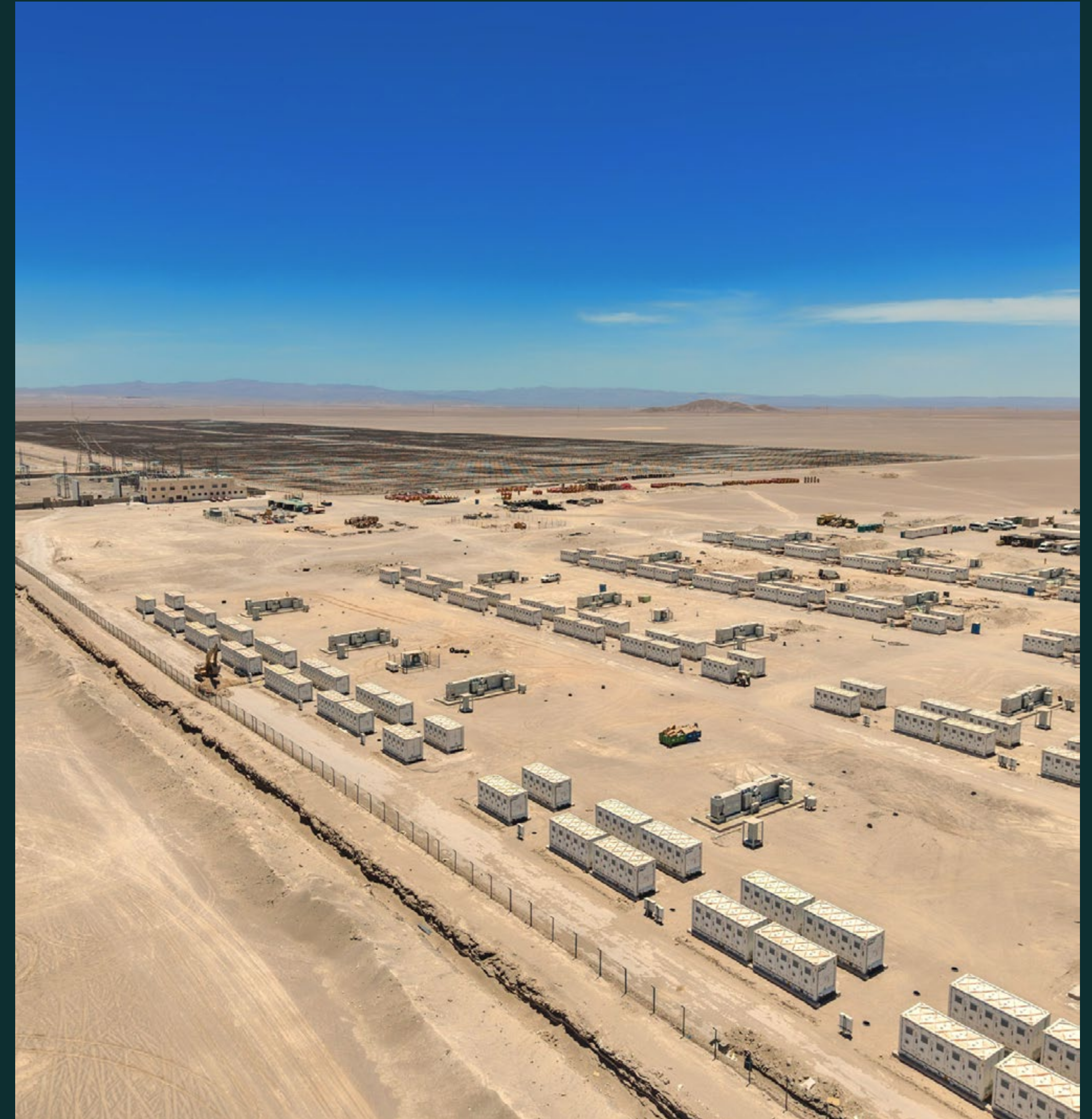
Elena 446 MW + 3.5 GWh hybrid plant, Chile
