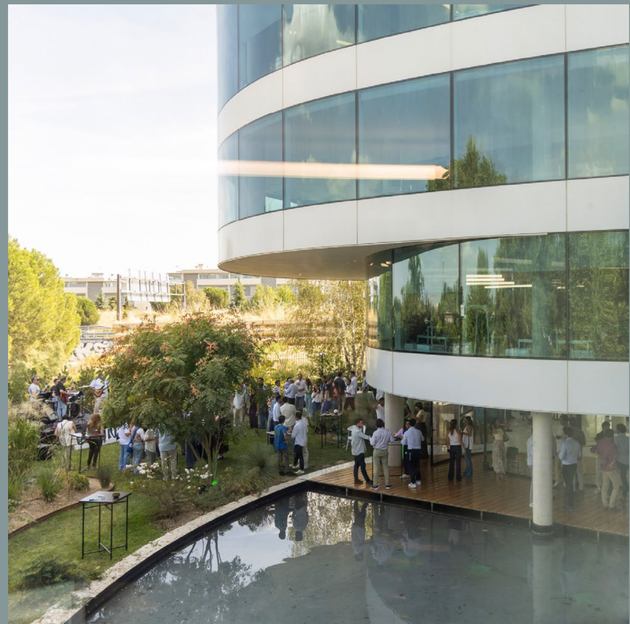
Greenergy headquarters, Madrid, Spain
